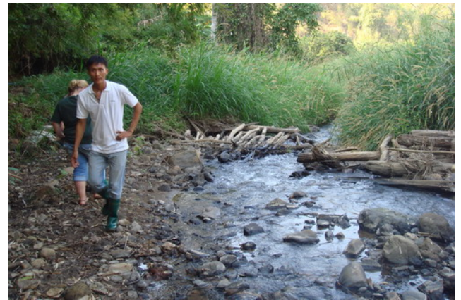
Damage that the dam received
