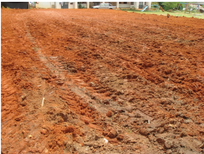
Leveling the land for the new Church building at Mae gone
